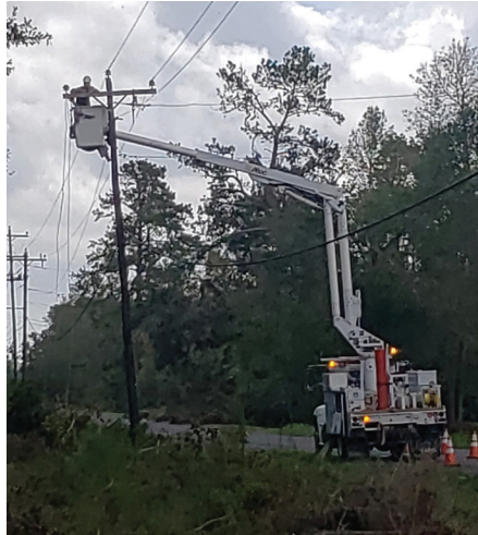
CMEC crews working in Louisiana
