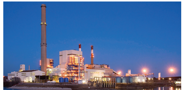
Thomas Hill Energy Center
